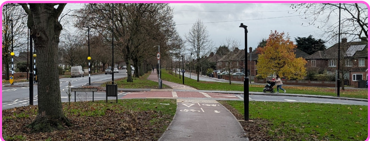
Figure 8: Cycle track low level lighting, Doncaster.
